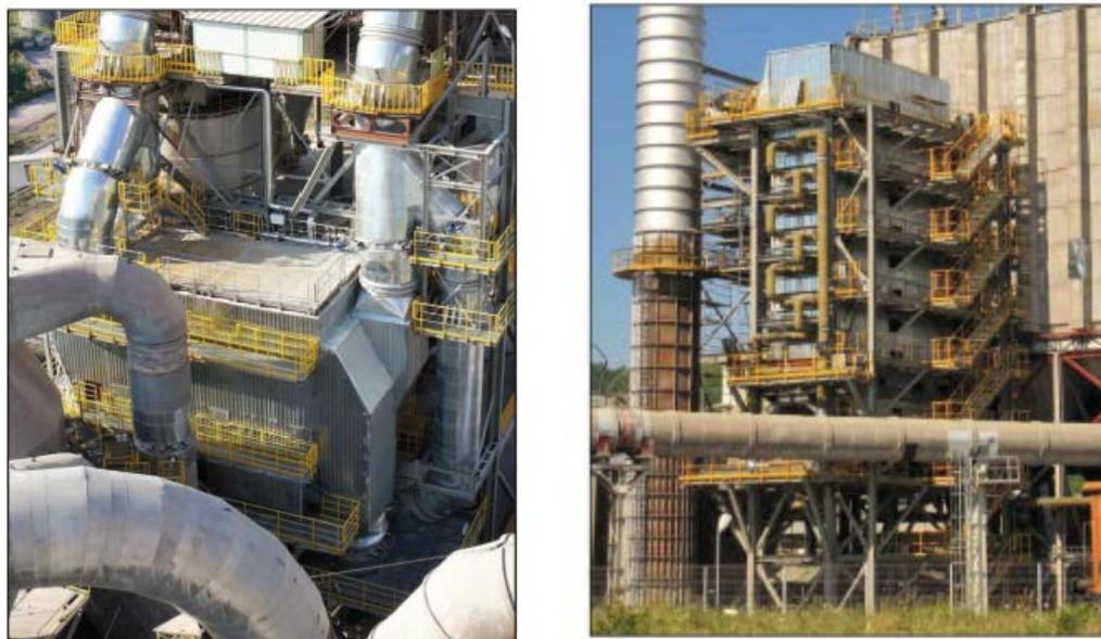
Figure 19. Preheater heat exchanger (left) and clinker cooler heat exchanger (right) [55].
